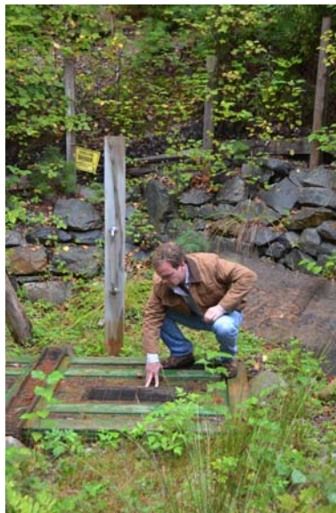
Director Chris Berlet at the entrance to the Gold Eagle ventilation shaft
